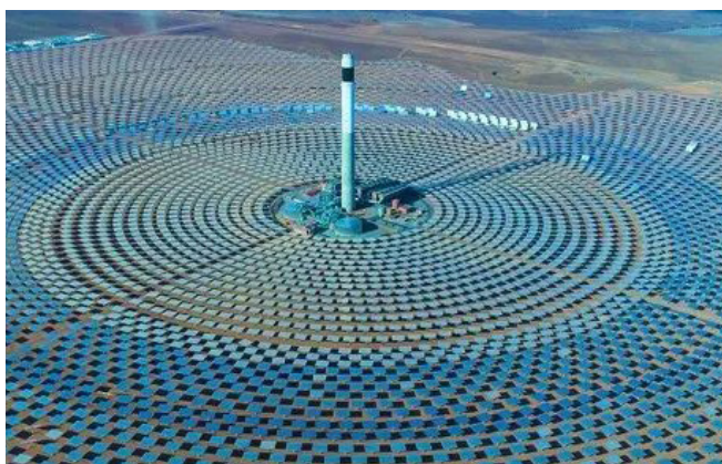
Figure 3-5-9 Eddy Current Tuned Mass Damper Application Case - Morocco Noor III Solar Tower
